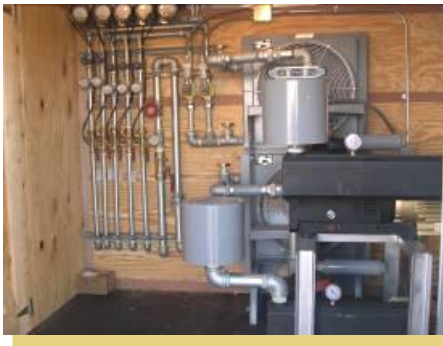
Trailer mounted claw sparge
